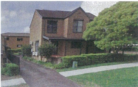
Photo 7: 69 and driveway to 69A Agincourt Rd
